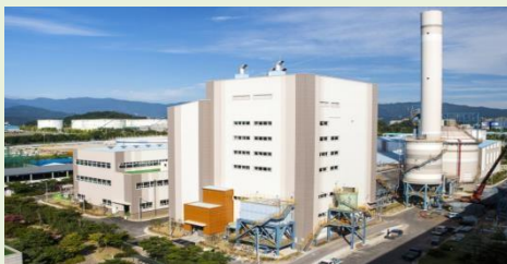
Picture 2 Biomass power generator
